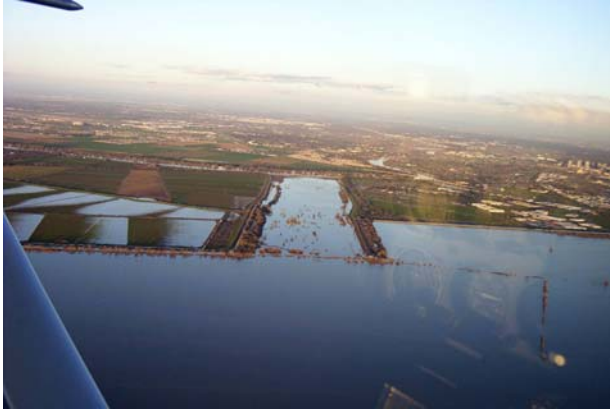
Figure 8, Sacramento Weir with Yolo Bypass in foreground, January 1997
