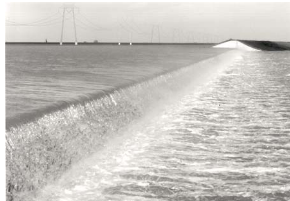
Figure 10, Cache Creek Settling Basin Weir, March 1995
