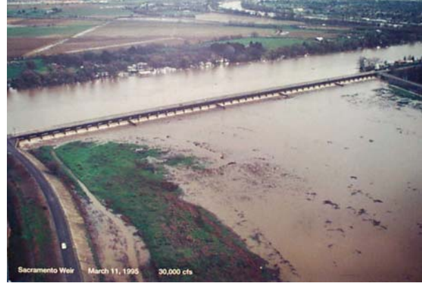
Figure 9, Sacramento Weir with American River in background, March 1995 (30,000 cfs)
